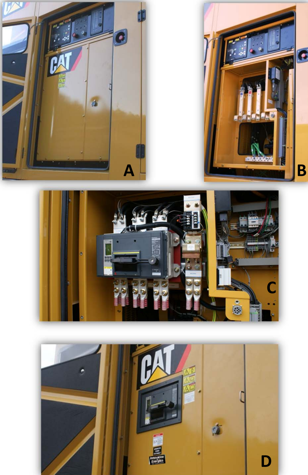
Fig. 5A-D, Before and After GENKIT Conversion, Typical CAT C27, Single CB
