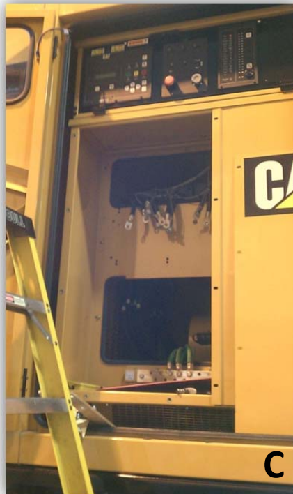
Fig. 6A-C, GENKIT Conversion, Typical CAT C27, Single CB
