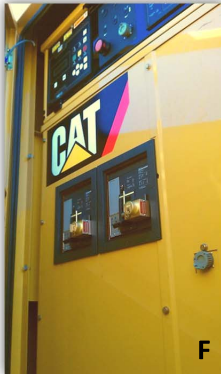
Fig. 6D-F, GENKIT Conversion, Typical CAT C27, Single CB
